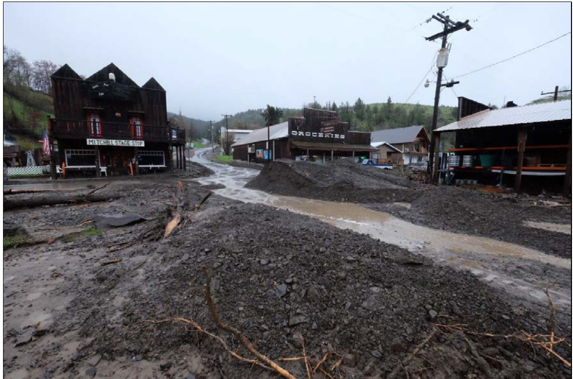
Downtown Mitchell, Oregon after the flash flood on April 20, 2019. Source: The Oregonian Newspaper.
